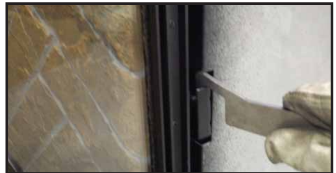
Figure 14.12. Securing Side Glass Clips
